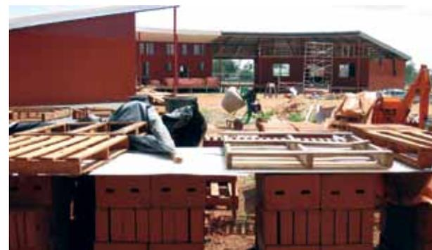
Fig 11.15 The building has been built using compressed earth bricks made on site by members of the local Aboriginal community.
